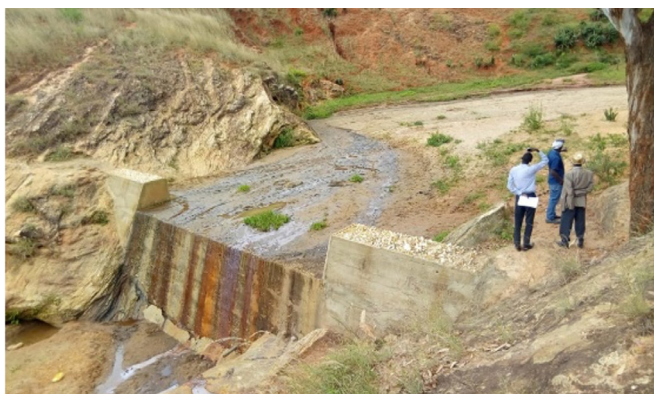
Kwa Lai sand dam, Makueni – functional © Adaptation Consortium
