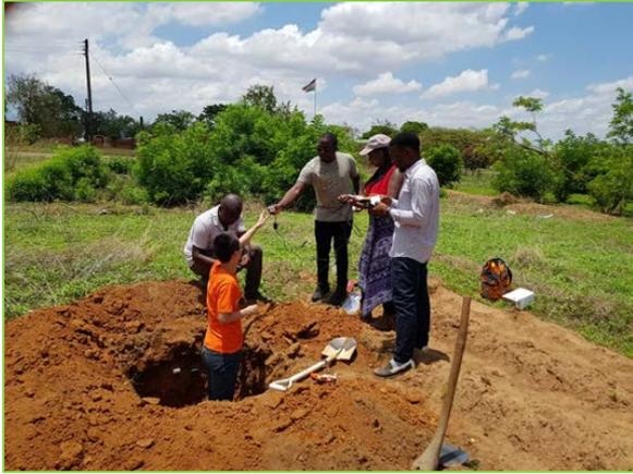
BRECCIA researchers installing Teros 10 soil moisture sensors at Namijiwa Vocational College in Malawi, where the experimental trial was being conducted
